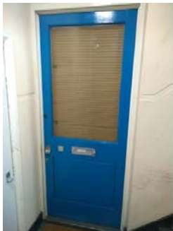
Typical Westbeeche front door with excessive glazing minimal locks
