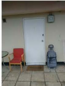
Typical Whymark front door – solid core door with minimal locks
